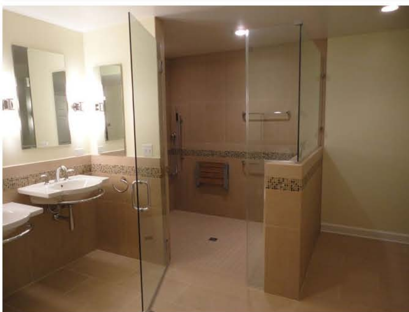
The curbless roll-in shower was designed for wheel-chair access. Photo courtesy of Glickman Design Build
