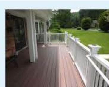
Photo contributed The new L-shaped front veranda wraps the home's northwest corner where it segues to a family grilling deck. Railing caps are fitted with night lights — perfect for evening entertaining.
