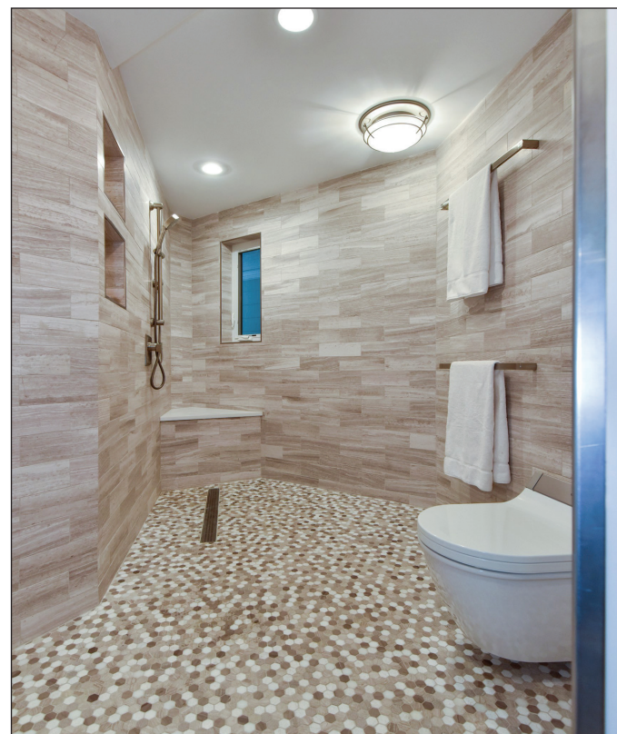
The 31 square foot shower incorporates the five foot turning radius needed for unfettered wheel-chair maneuverability.
