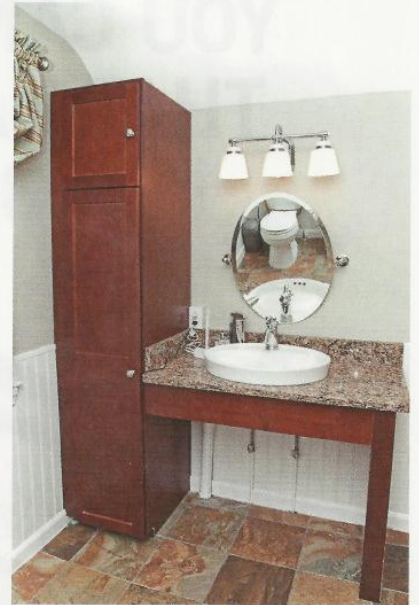
Glickman Design Build installed an accessible vanity so the homeowner can position her wheelchair under the counter while ensuring her legs aren't burned on hot pipes.
