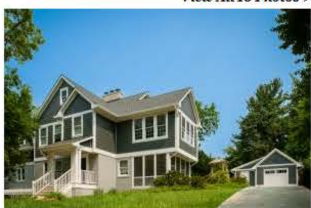
A home in Bethesda, Md. gets a top-to-bottom makeover and a second floor addition. See the transformation.
